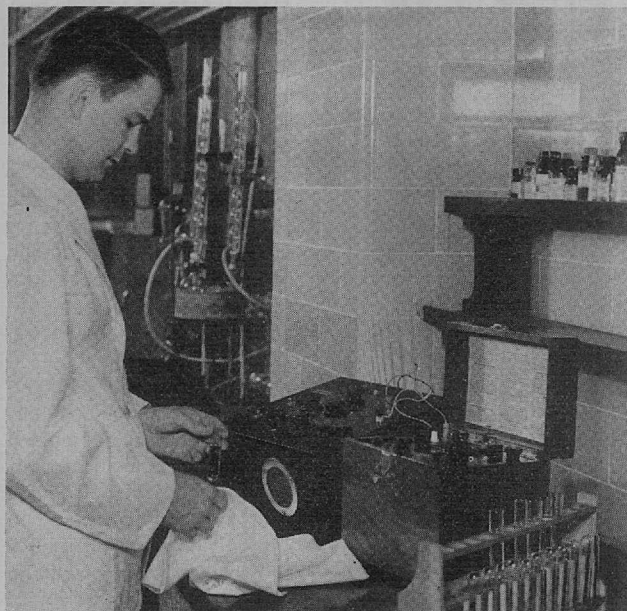
FIGURE 63. DOUBLE MONOCHROMETER SPECTROPHOTOMETER IN CHEMICAL RESEARCH
